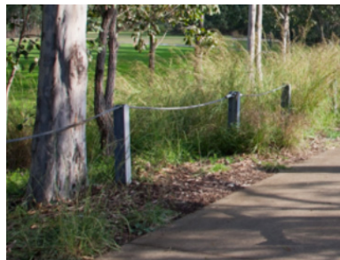
Exposed aggregate concrete threshold
