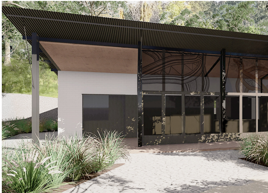
Figure 3.45 Kui Kiosk – view of at grade access to deck from carpark
