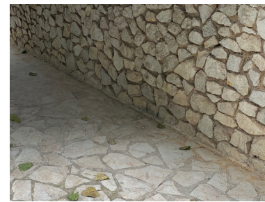
Stone clad walling
