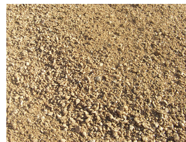
Stabilised gravel pavement
