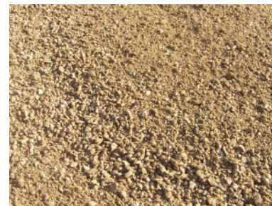
Stabilised gravel pavement
