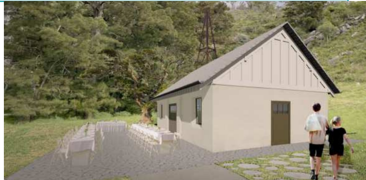
Figure 3.49 Power House (ISP) view
