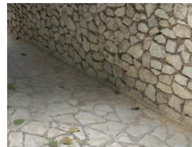
Stone clad walling
