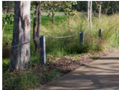
Exposed aggregate concrete threshold
