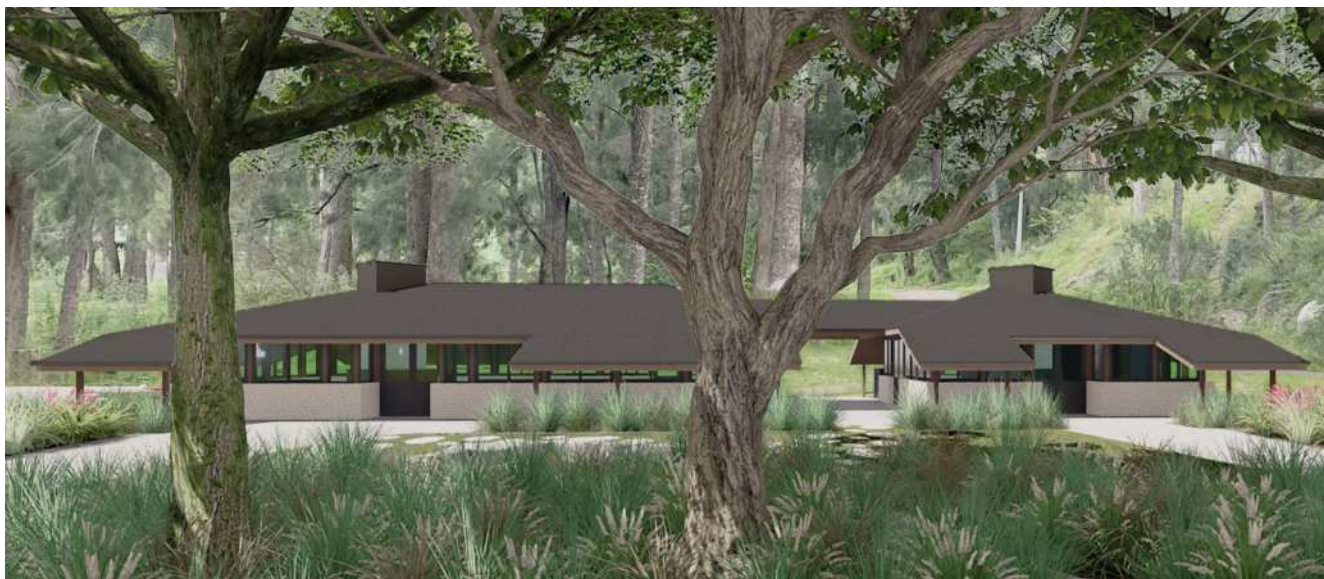
Figure 3.9 Barmah ISP refurbishment front view – roofline opened up at primary entries.
